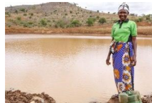
The Musosya dam was first cleared of silt and debris and is now collecting water.
